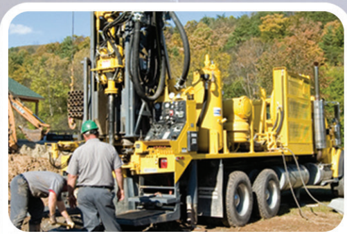
TH 60 WATER WELL RIG
